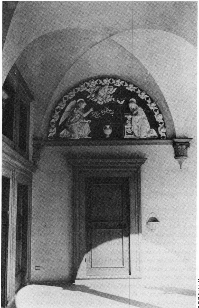
Interior, Hospital of the Innocents , built by Brunelleschi, 1421.
